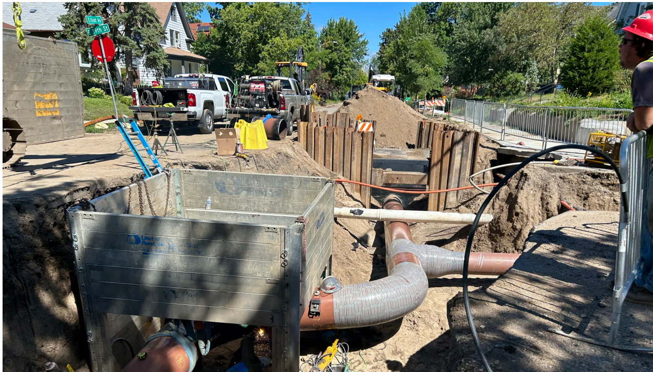
Utility workers updating a gas main in South Minneapolis
