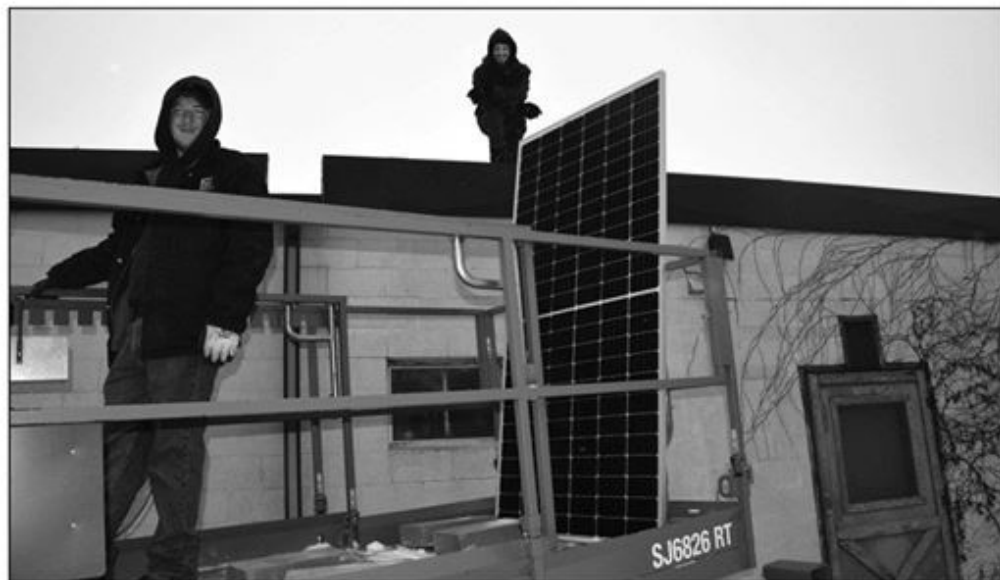
Mike and Mike, installers for MnSolar, lifted one of the 56 panels in place on the top of the Kerkhoven Banner building. The project will convert sunshine
